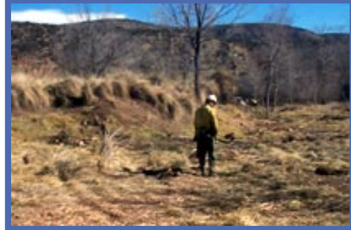
BLM crews used chainsaws to clear trees.
