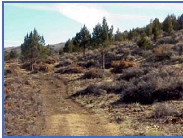
Completed section of the fuel break.
