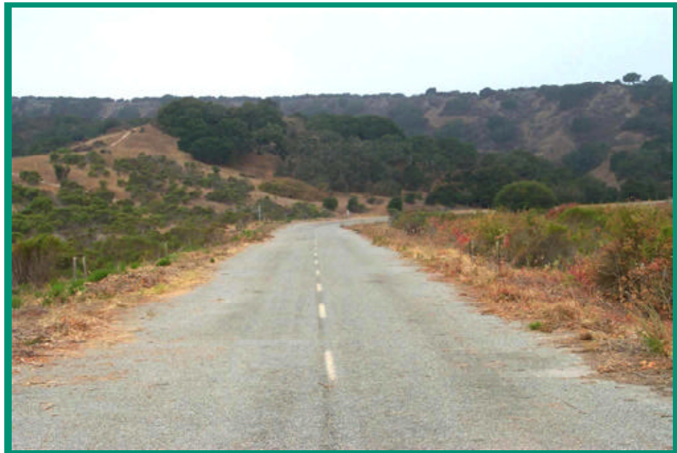
Same section of the road following treatment.
