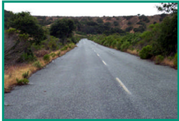
Section of Reservation Road before being treated.
