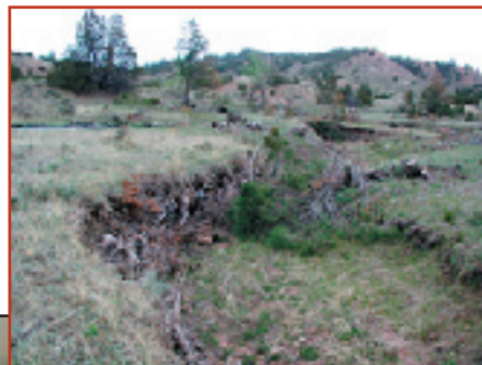
View of a revetment in the stream channel.
