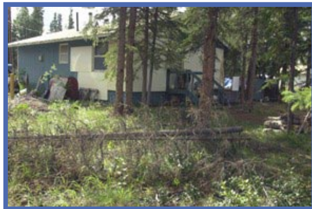
Homes and office at risk to wildland fire.
