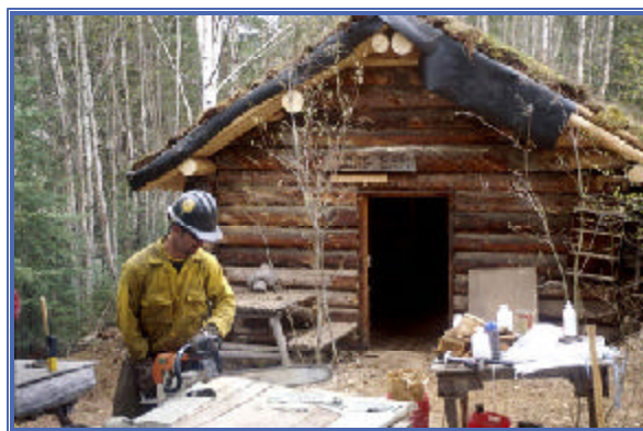
A firefighter works to restore the cabin door.
