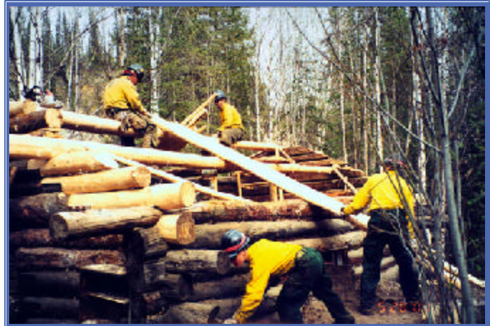
Alaska Fire Service fire crews install a new roof.
