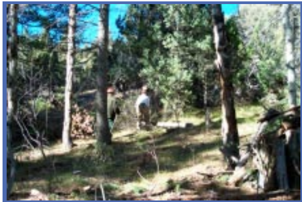
Crews cut, clear and pile brush and trees for lava ranches project.
