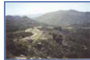
Completed fuel break outside community of Poppet Flats.
