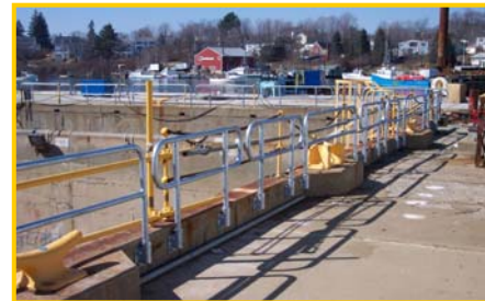
Guardrails around the perimeter of PNS dry-dock
