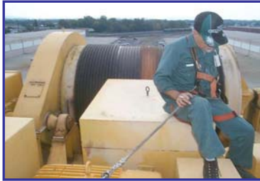
One anchor point for fall arrest gear resulted in very limited working area
