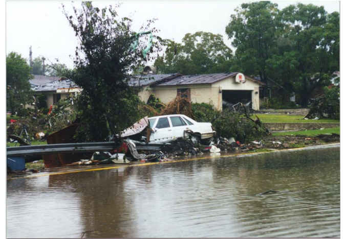
This home located along the Guadalupe River in New Braunfels is still standing although the roofing has been stripped away by floodwaters. Across the street, 10 brick homes were destroyed after being swept clean from the concrete slabs by floodwaters. Flood depths in this area were estimated to be 25 feet above normal flow--greater than 500-year event levels.
