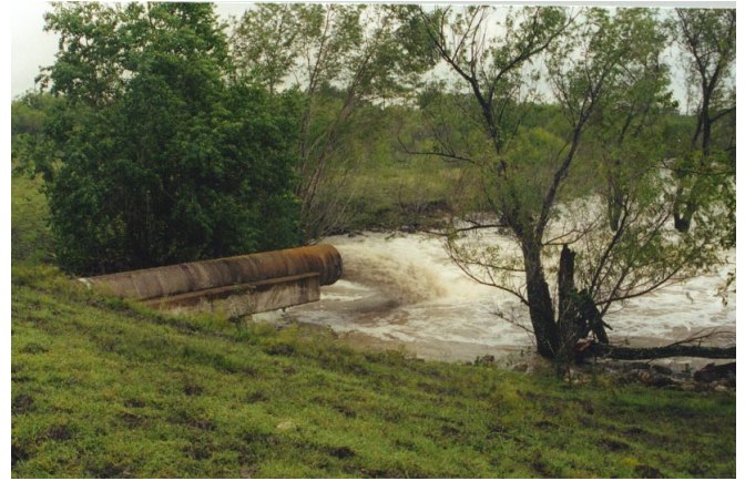
Principal spillway flow of Plum Creek floodwater retarding structure. Flows will continue for up to 10 days after the rainfall ceases. This slow release of the captured storm runoff prevents or greatly reduces downstream flooding.
