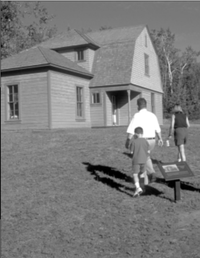
Two scale models of these non-commissioned officers' quarters at Ft. Egbert National Historic Site at Eagle were created to publicize the Save America's Treasures program. One model joined replicas of other historic properties at a special Christmas display at the White House. The other remained in Alaska. The Eagle Historical Society hopes to raise $50,000 to match an equal amount available through a challenge grant to rehabilitate the quarters shown here. Photo by Anne Jeffery.
