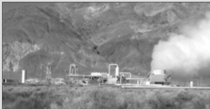
Caithness Power, Inc., geothermal power plant in Dixie Valley, Nevada.
