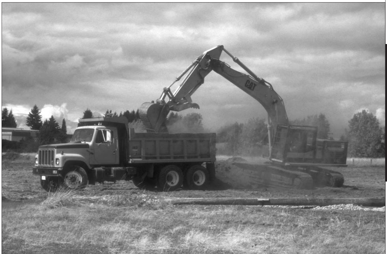
Road maintenance crew at work in Oregon.
