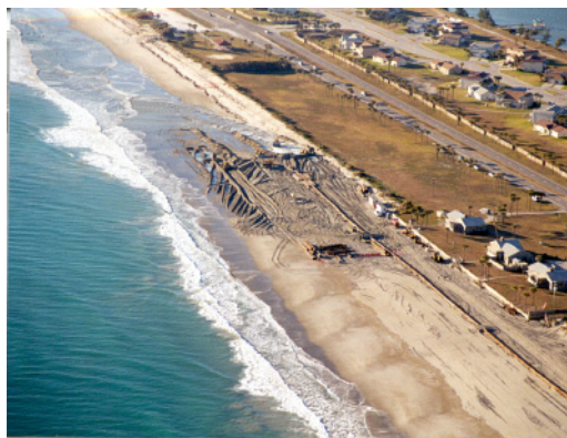
Beach Nourishment Project at Patrick Air Force Base, Florida 2001.
