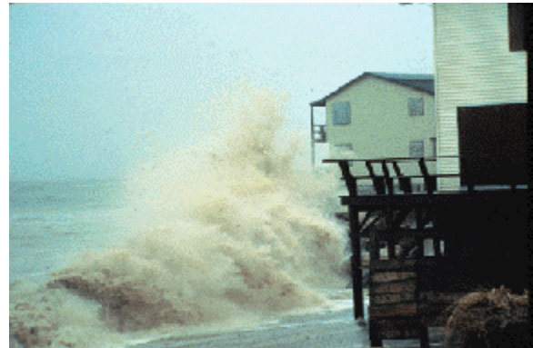
Home threatened by coastal erosion.
