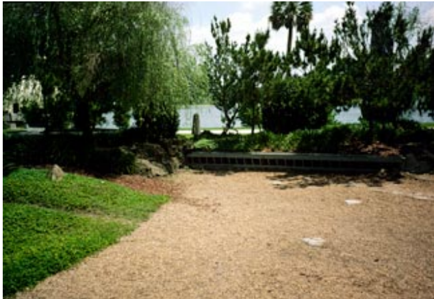
Another management method is the use of dry-retention basins, which can be incorporated into the landscape of lakeside parks. Shown above is a dry-retention basin near Lake Eola in downtown Orlando, Florida.
