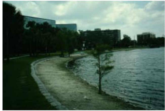
The drawdown or lowering of the water level in an urban lake sometimes is used to improve water quality by exposing the lake bottom for sediments to become oxygenated. Here, Lake Eola in downtown Orlando is shown, August 1994.
