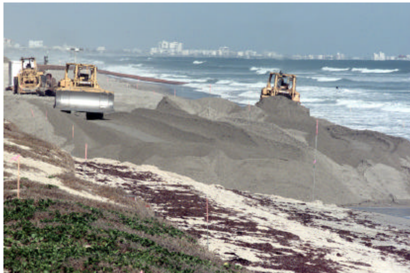
OCS sand is placed on Patrick Air Force Base, Florida
