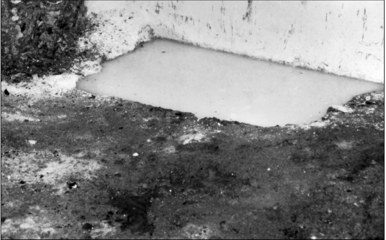
Figure 7.—Freshly prepared gel in pit in mine floor.
