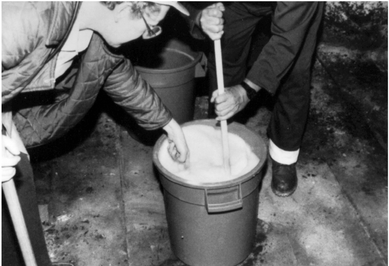
Figure 4.—Mixing of all the ingredients with a wooden paddle to form a gel.
