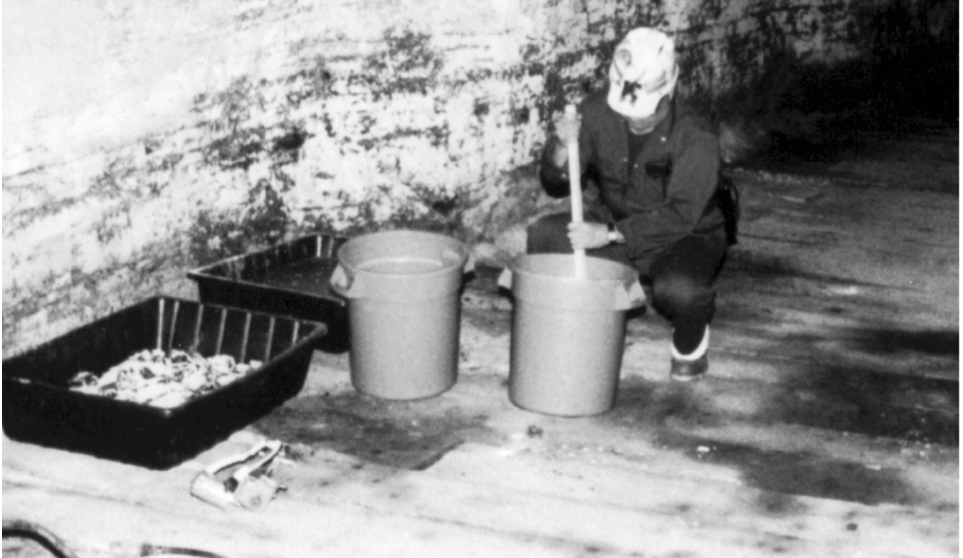
Figure 3.—Two plastic tubs with coal pieces and rock dust are being placed next to the coal rib while dry ingredients with ethylene glycol are being mixed prior to the addition of water.
