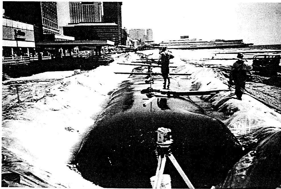
Figure 1. Construction of the geotextile tube in front of the Atlantic City, NJ, boardwalk
