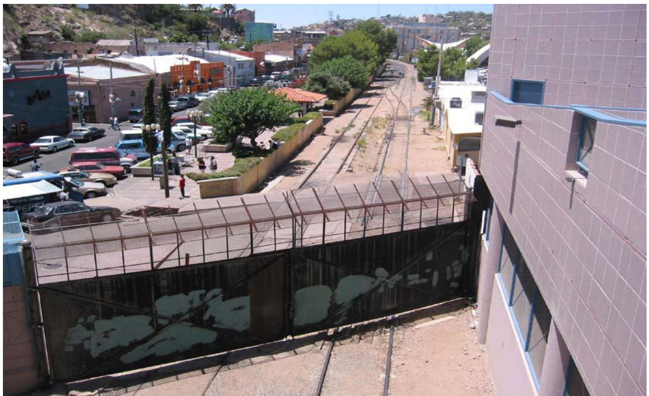
Train tracks cut through the border (gateway) between the U.S. and Mexico and the downtown area of Nogales, Sonora and Nogales, Arizona. Nogales POE. June 2003.
