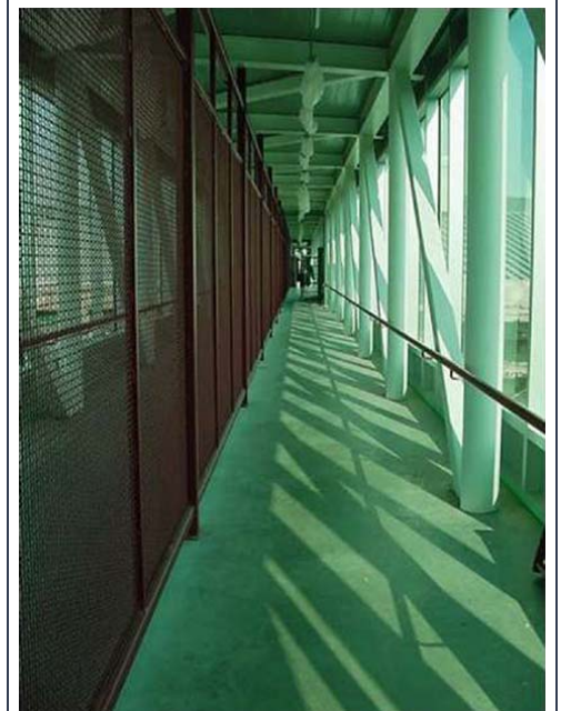
This walkway above the main road at the shared facility in Sweetgrass, MT marks the international border (red chain link fence) between the U.S. and Canada. Sweetgrass POE
