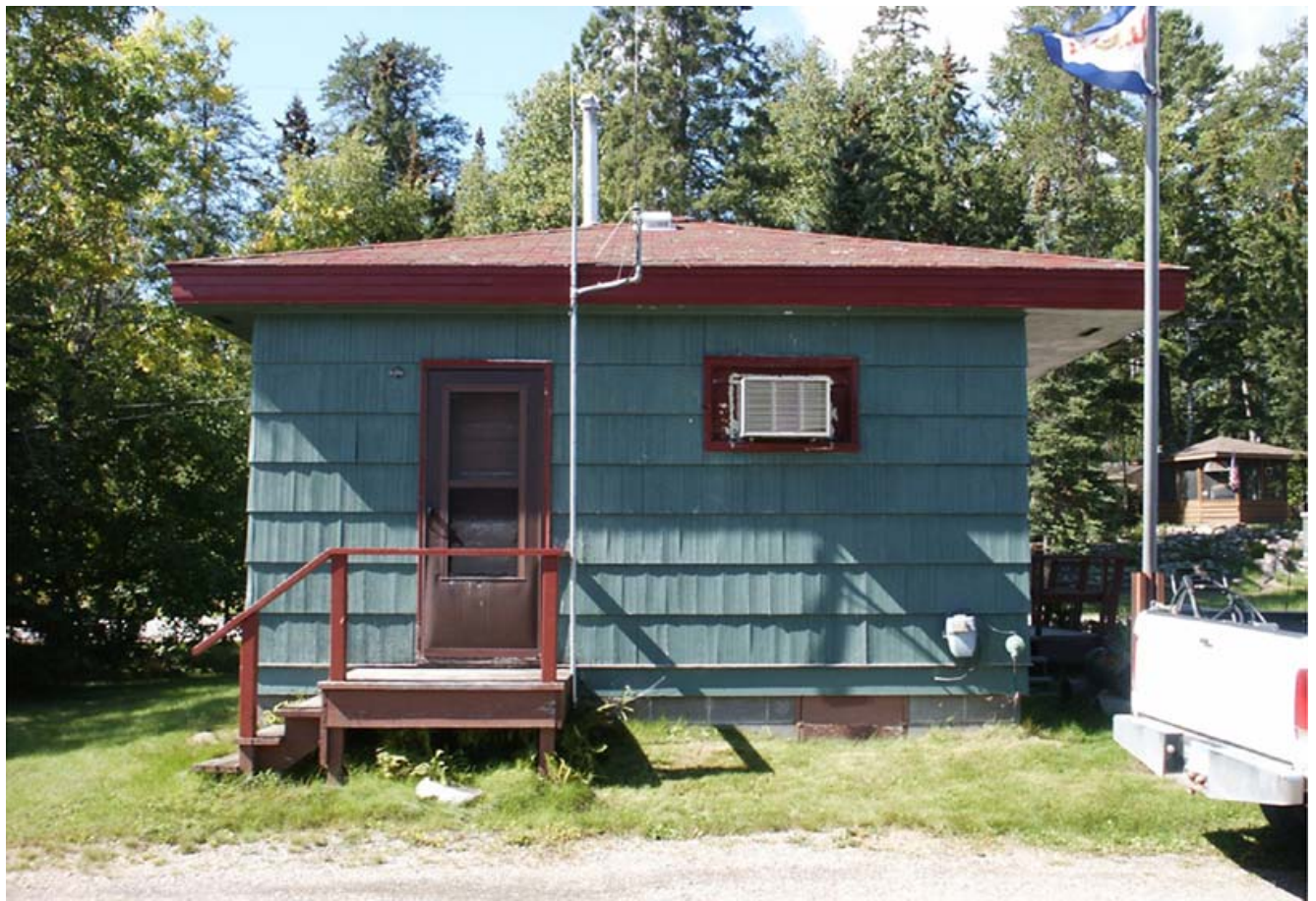
The main building at the Crane Lake POE. Crane Lake, MN.
