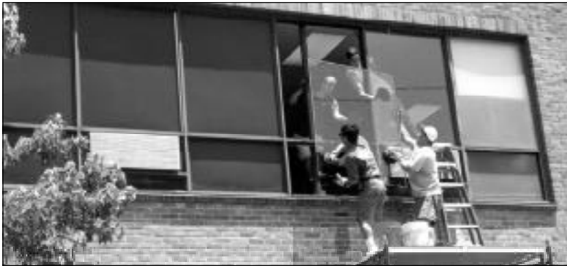
By replacing the existing windows, this Rebuild America partnership school improved indoor comfort while reducing winter heating requirements.
