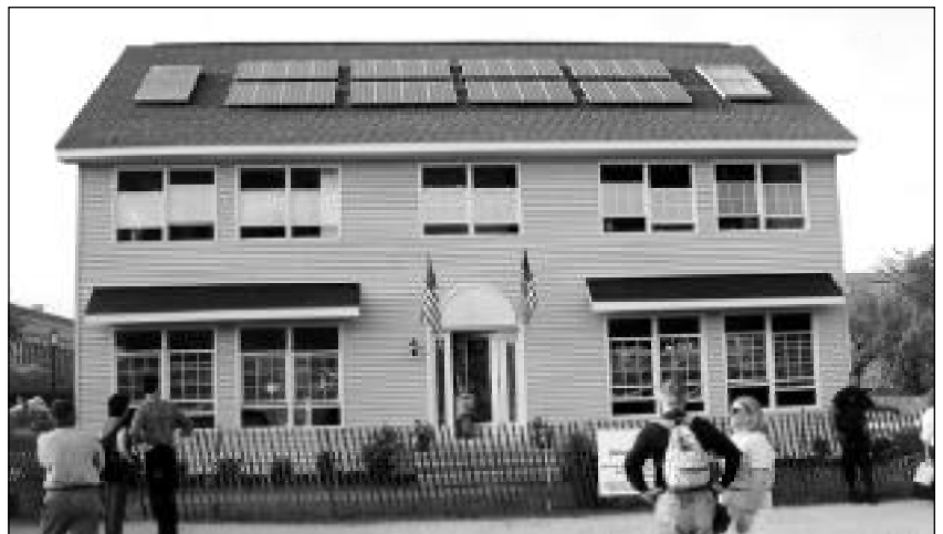
Solar water heaters are simple devices that capture the sun's energy to heat water for ordinary use. They are often piped directly into systems with conventional water heaters, lowering your energy costs while still providing hot water on overcast days
