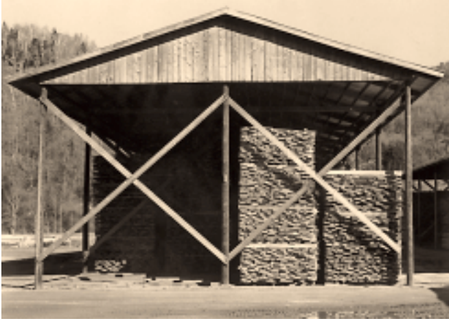
Figure 5.3—Air drying pole shed for hardwood.
