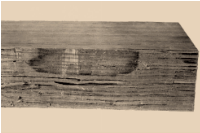
Figure 9.2—Dirt and stain inside a check, a certain indicator that the check was open during air drying.
