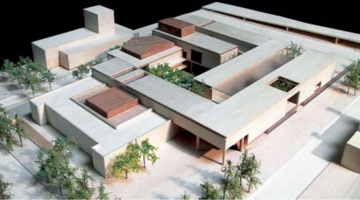
Project model, "loft" spaces that house the making and presentation of art "rotate" around the amphitheater
