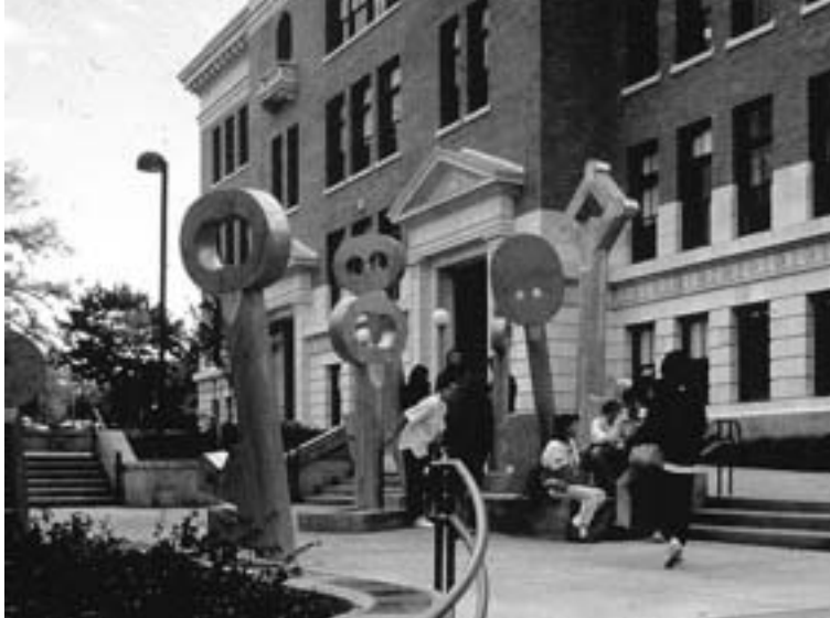
The Franklin High School in Seattle was built in 1912 but renovated to meet state-of-the-art standards in 1990.
