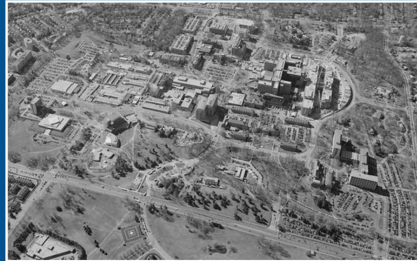
Aerial view of the NIH Campus in Bethesda, Maryland
