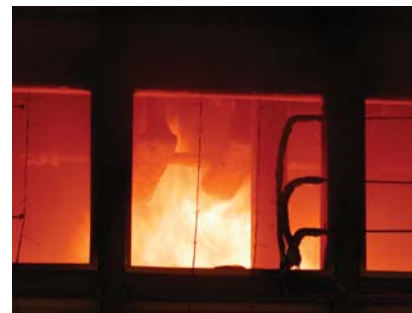
View of fire compartment from air exhaust outlet several minutes after the start of a fire test. Note the flame impingement on the steel trusses and bar
