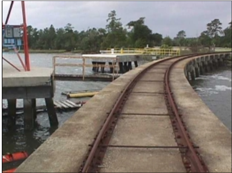
View showing access to tower base at NWS Charleston
