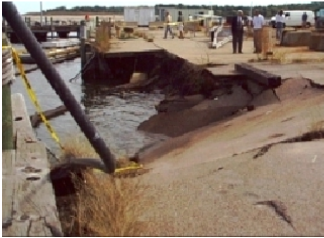
Collapsed portion of Pier 172
