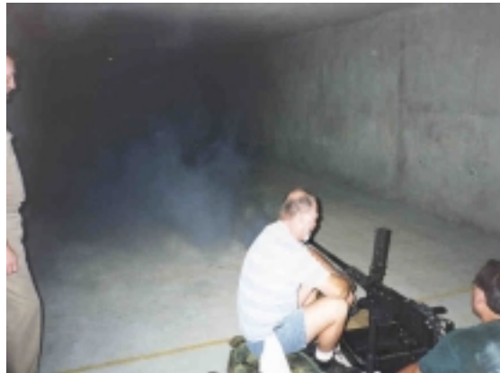
Smoke test is conducted at indoor firing range to ensure adequate exhaust ventilation.
