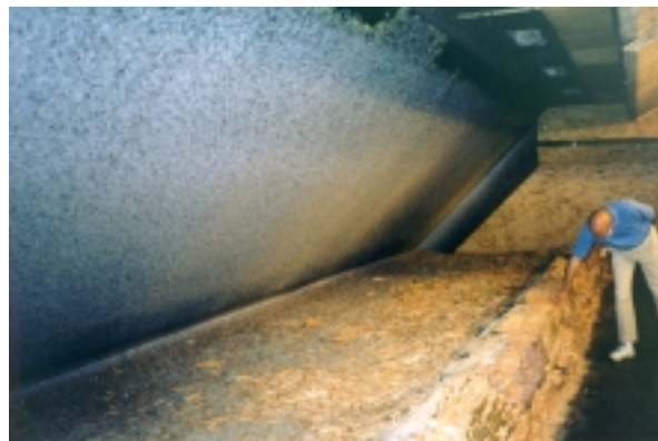
Plate and sandpit bullet stops are undesirable because they require high-level maintenance.
