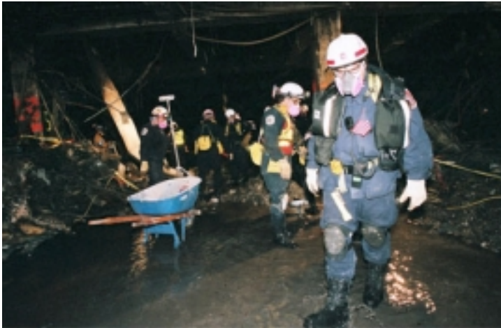
Many areas of clean up site lacked electrical power and lighting
