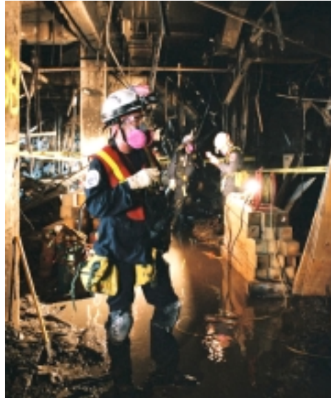
Clean up crews wore full-body protection and respirators
