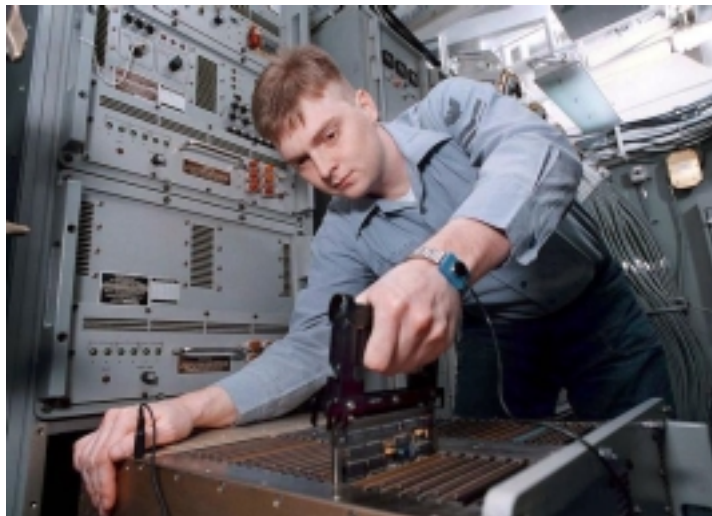
Performing maintenance on electronic communications equipment.
