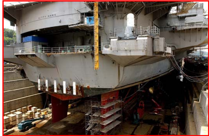
USS Kitty Hawk (CV 63) undergoing repairs in dry dock.
