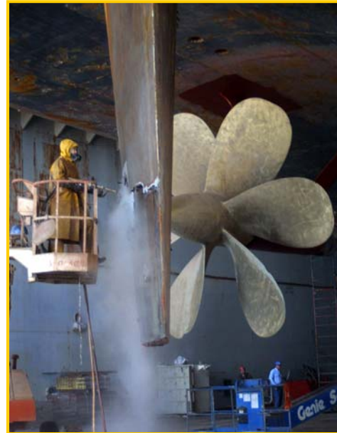
In dry dock, worker hydro-blasts Amphibious Ship propeller for preservation.
