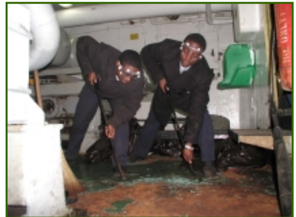
Two of the USS John F. Kennedy's crew members removing floor tiles in the launch catapult room during the ship's ESRA.
