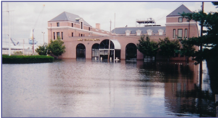
Naval Reserve Center Baltimore was flooded due to a storm surge during Hurricane Isabel
