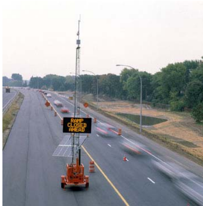
Figure 5-1 Portable Traffic Control Devices can assist with Work Zone Activities.
