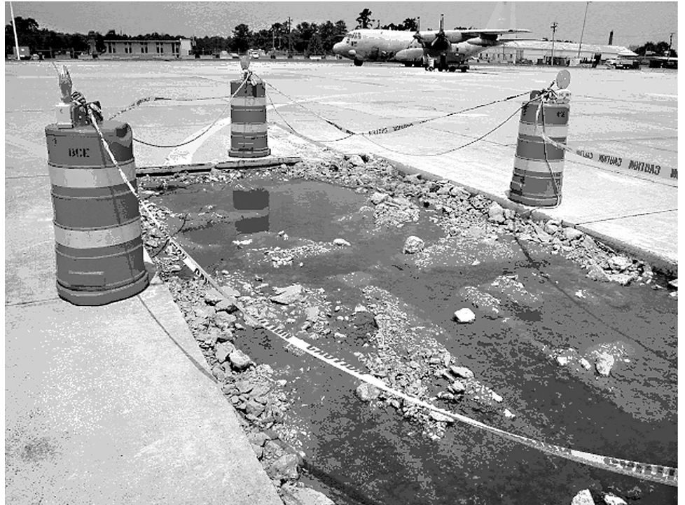
Figure 6: Parking Runway Ramp at Dobbins Air Reserve Base, Georgia (August 2002)
