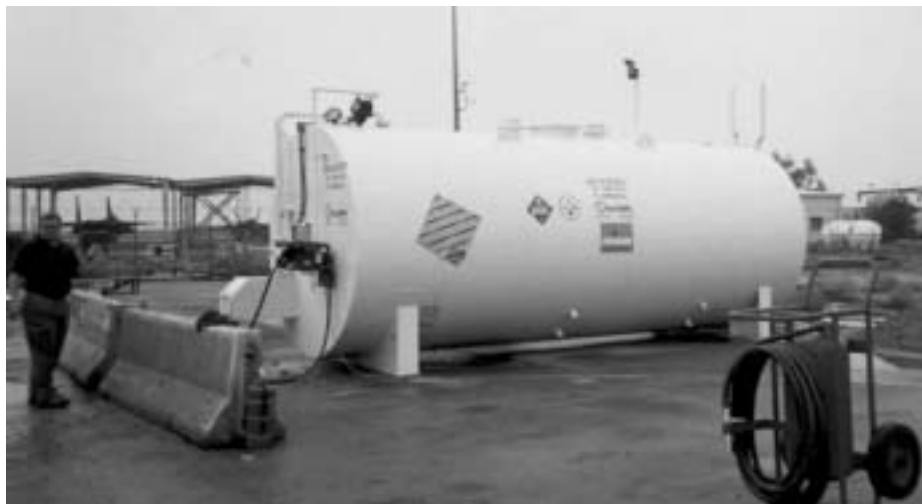
Jeff Feltner, DESC-ME quality manager, inspects an above ground tank.
