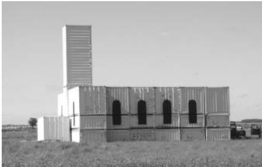
One of the buildings made from the containers provided through DRMS in the mock city used for anti-terrorism training by military services. (Photo courtesy of DRMO Norfolk)
