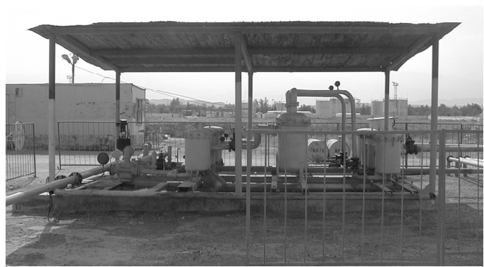
Inspected fuel pit in Ashgabat.
