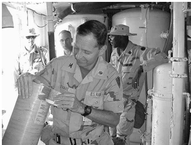
Filters for Purity – Col. Emmet O'Hare, DSCT Commander for Exercise Bright Star, examines a filter element for a Reverse Osmosis Water Purification Unit. DLA is responsible for repair parts for the units, thereby ensuring the availability of fresh water in theater. The filter is cut apart to show the many layers of filter elements and how they act to purify the water and remove salt and other impurities. (Photo by Gunnery Sgt. Ruben Ellis)
