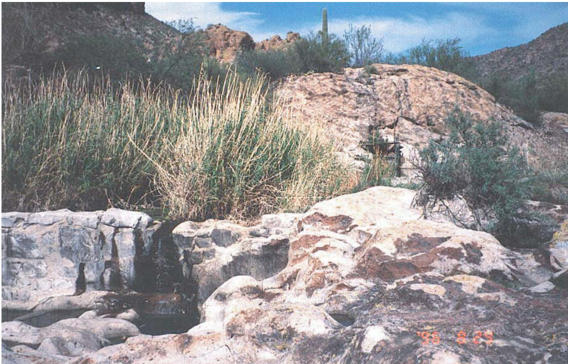
Figure 27. View looking upstream at gaging station from left bank, Tortilla Creek at Tortilla Flat, Arizona.
