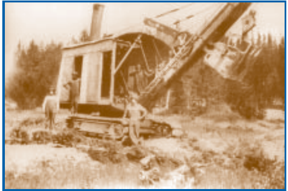
Drag Line or Steam Shovel Dredge in Florence Basin
