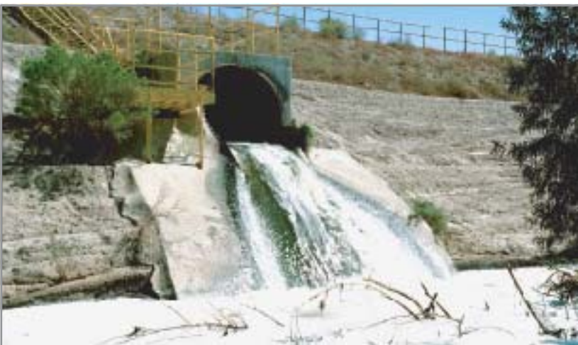
Figure 5. Effluent release to the Santa Cruz River from the Roger Road wastewater-treatment plant, near Tucson, Arizona.
