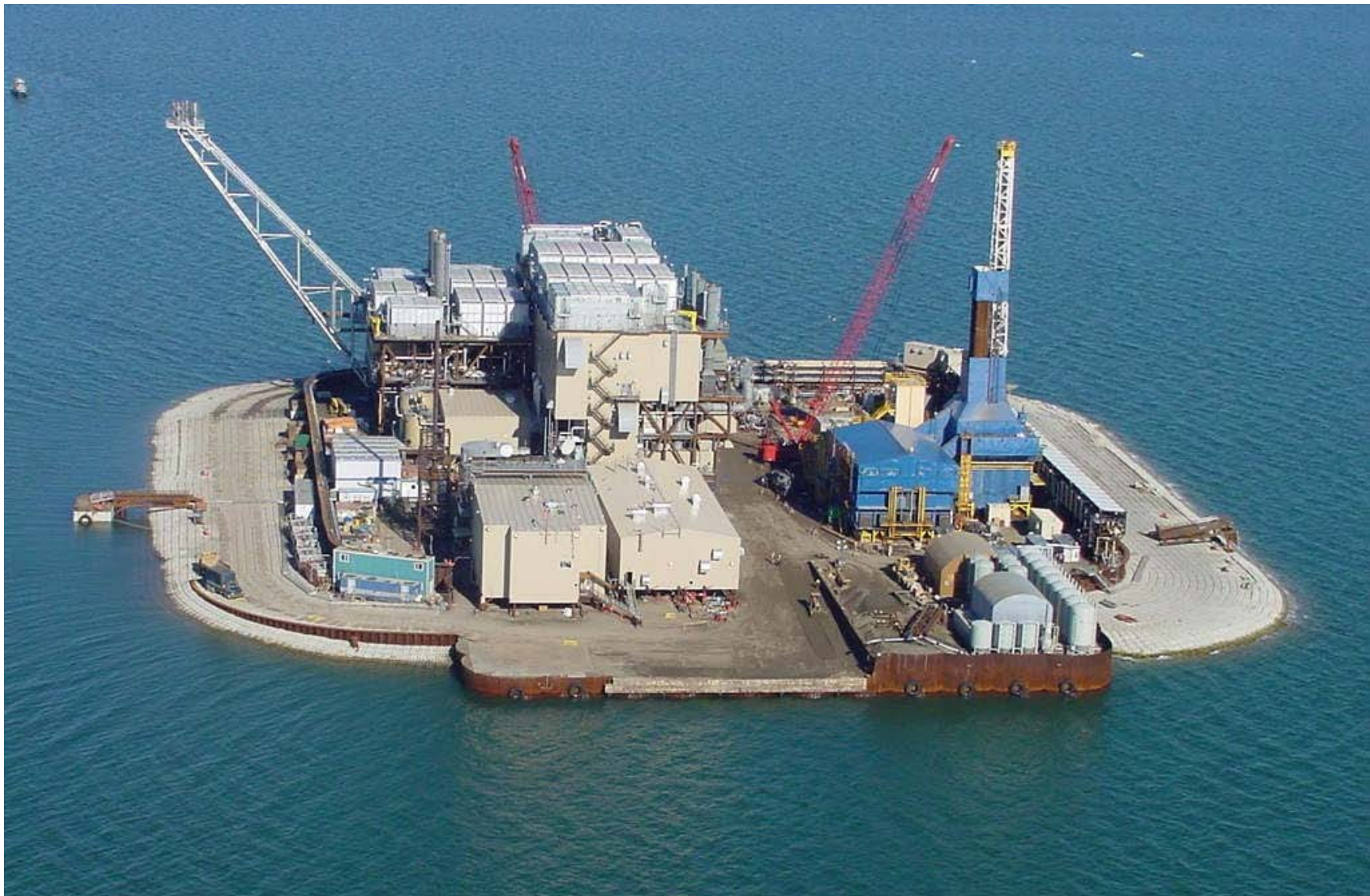
Fig. 3 Northstar Island looking north, September 2001. Production started in November 2001.
