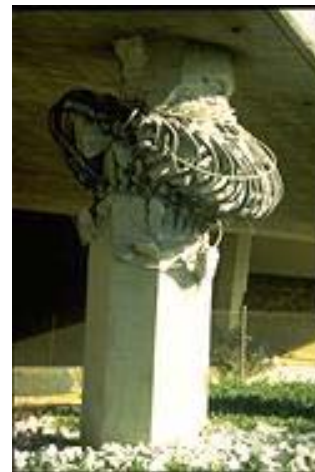
Highway 118/Bull Creek Bridge
