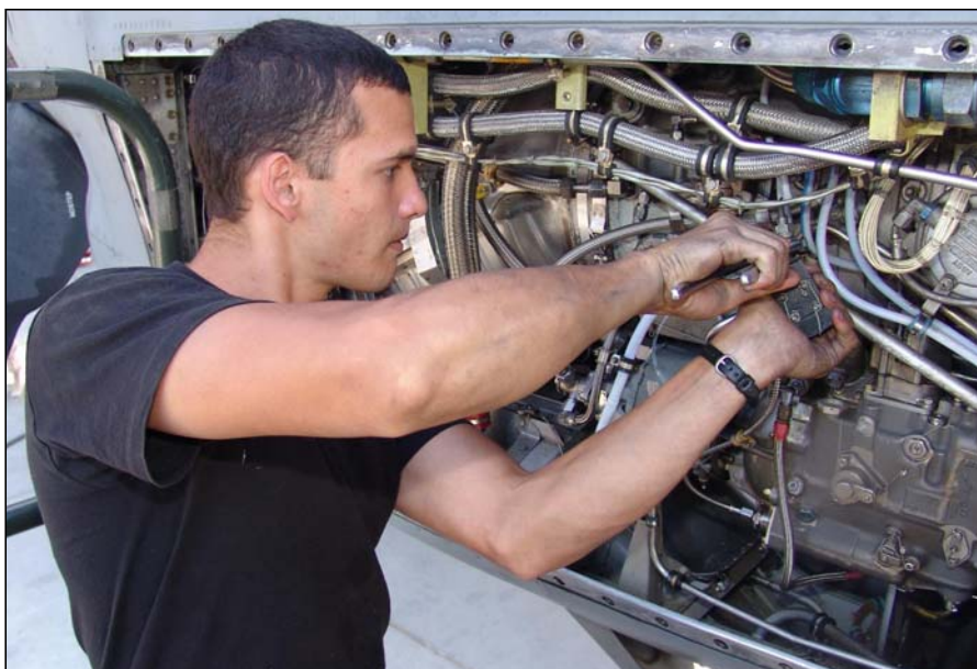
Airman Torres tightens a cannon plug on an engine fuel control assembly.
