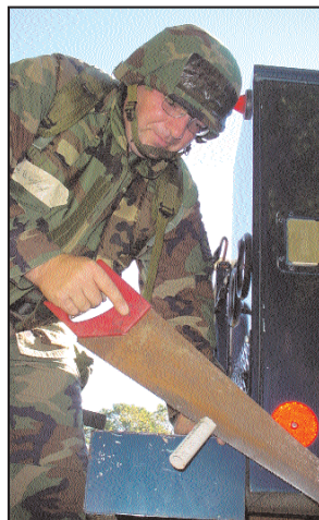
Tech Sgt. Ronald Burgdorf cuts a pipe to repair broken water pipes.
