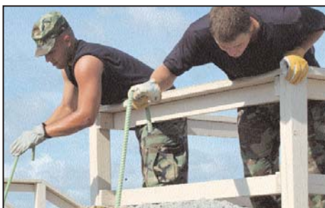
Staff Sgt. Jason Knecht, 45th Medical Support Squadron, left, and Airman 1st Class Mariuz Targonski, 45th Comptroller Squadron work sand down into a sandbagger machine.
