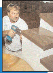
Seaside Chapel undergoes major renovations
