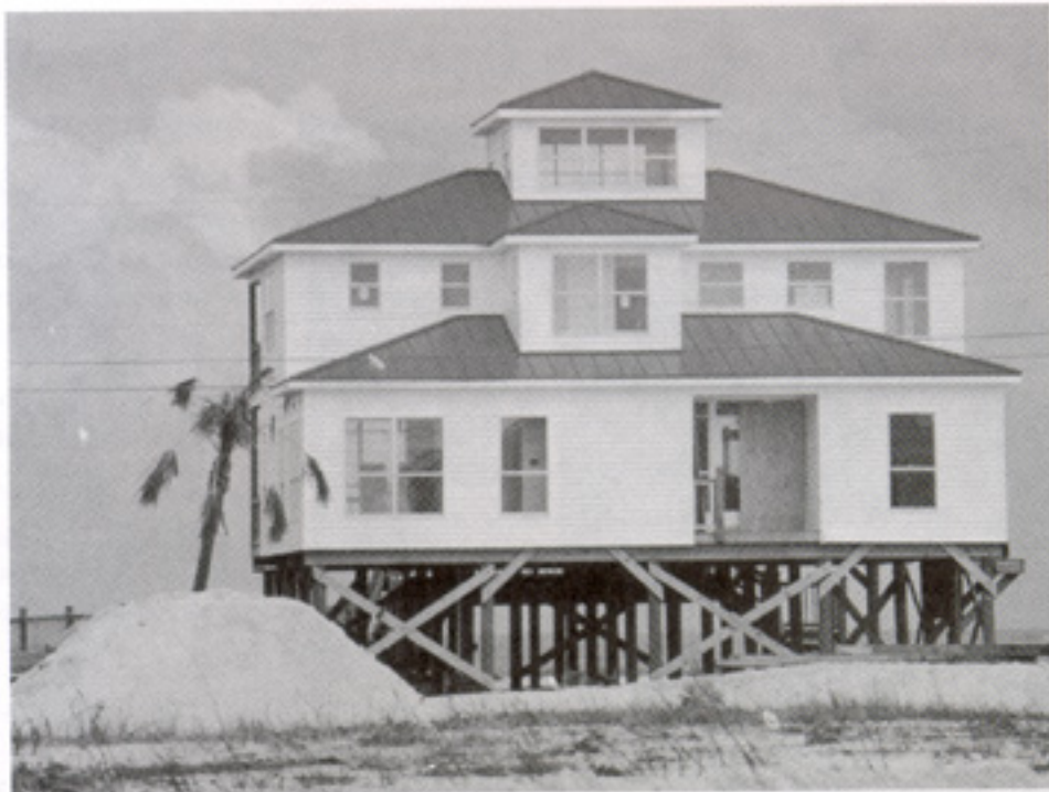
This home was elevated to prevent damage from future storms and flooding. Elevation can reduce flood insurance premiums significantly.
