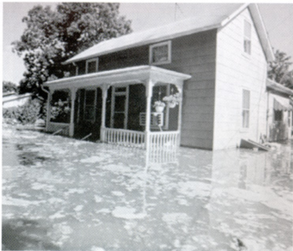
Floodwater causes mold and mildew as well as germs and bacteria.
