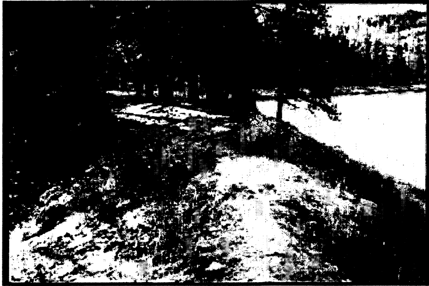
Photo 2 Helena NF- Park Lake Dam-Large Trees on Embankment
