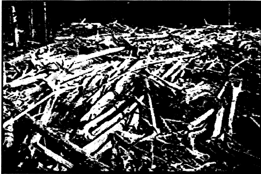
Photo 6 Beaverhead NF-Pear Lake Dam-Excess Tree Debris on Dam
