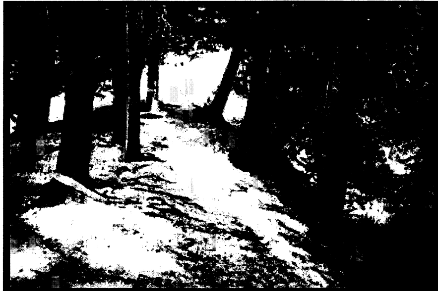
Photo 3 Helena NF-Park Lake Dam-Large Trees on Embankment
