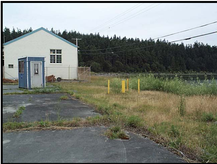
Operable Unit 4, Area 41. View of Area 41 that shows existing ground surface and vegetation. Sea wall and Oak Harbor are present to the right in the photograph.
