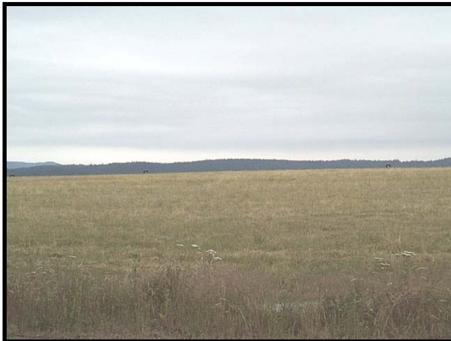
Operable Unit 1, Area 6. View of Area 6 landfill. Area 6 landfill is covered with a minimum functional geosynthetic cap with a vegetative cover. Note passive landfill gas vents in background.
