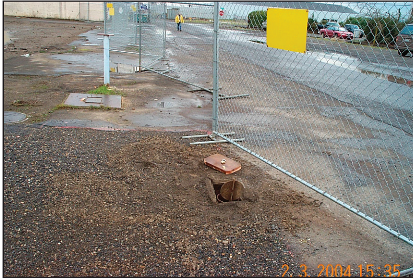
Well B85-3 looking south. Well in foreground with cover removed.
