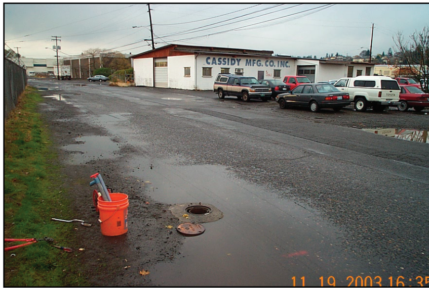
Well B85-4. Facing W.
