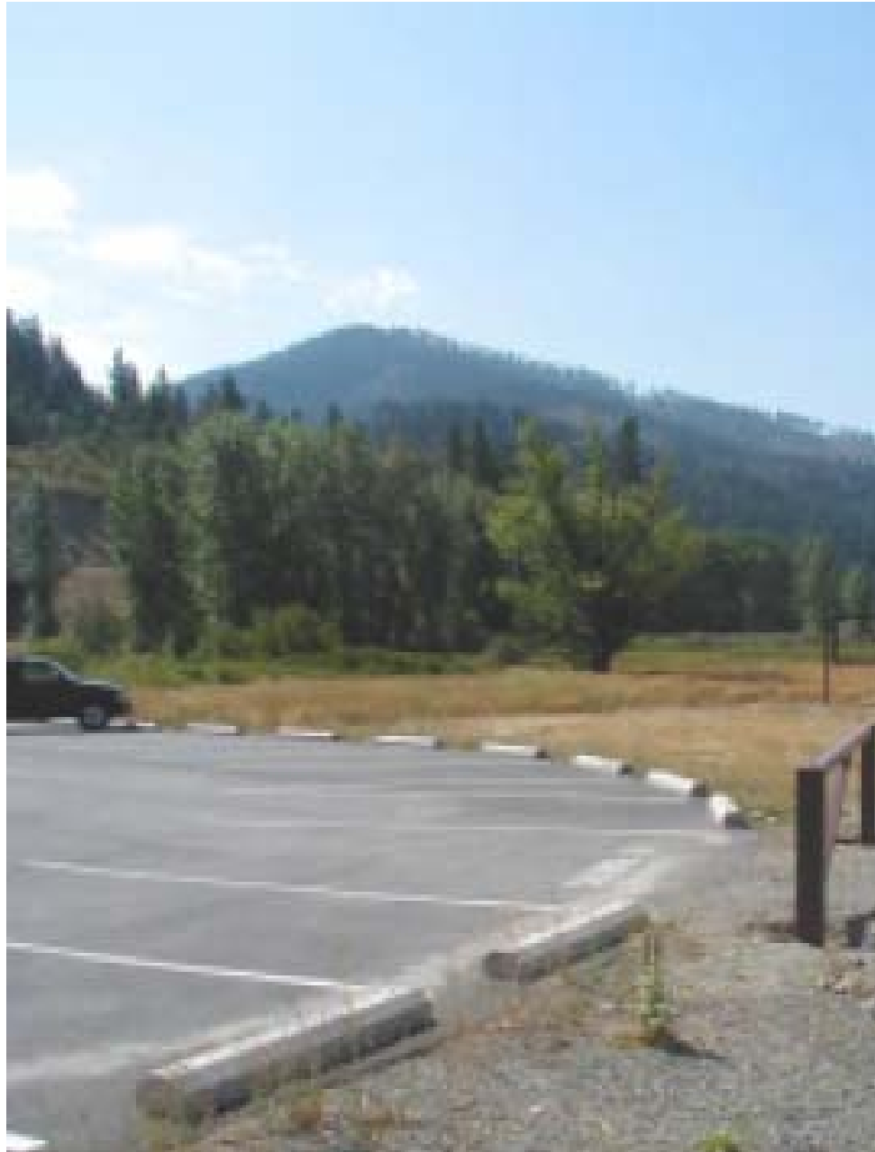
Highway 3/Trail of the Coeur d'Alene (Black Rock Trailhead) parking lot looking westward. Area to be capped is adjacent to the parking lot to the right.
