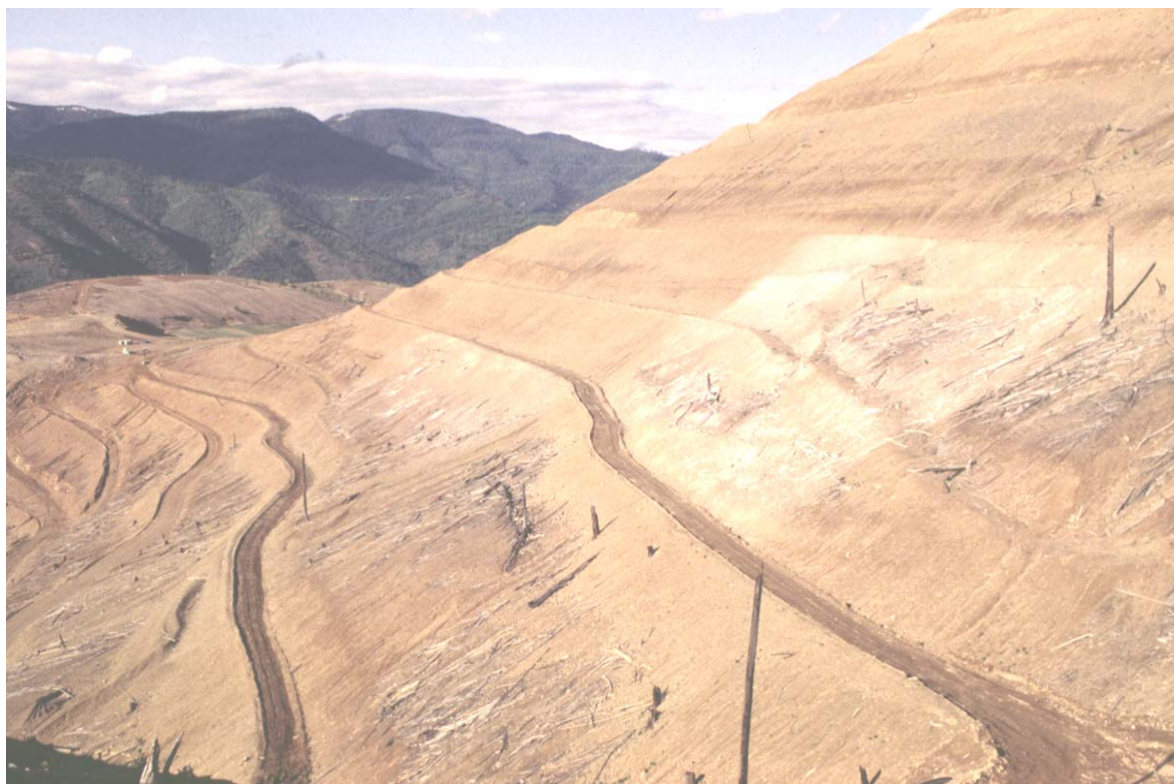
Figure 1. Pre-treatment hillsides environment in Government Gulch. Note construction of terrace benches spaced approximately 30 m apart. Steep slopes, exceeding 30 degrees (58 percent) and extending to over 500 meters in many places, dominate the site. Combined with extensive soil erosion, acidic reaction, and even steeper cut and fill slopes, the hillsides landscape is a difficult restoration challenge (1997).
