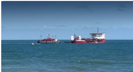
Offshore Dredge used to pump sand to the Patrick Air Force Base, Florida 2001.
